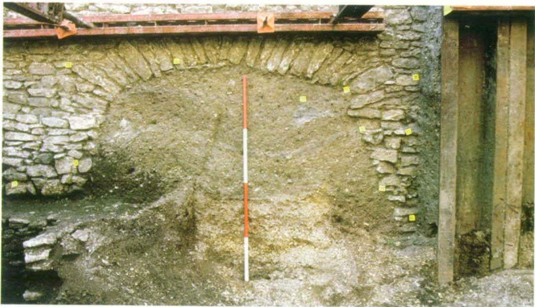
Plate XIII. Relieving arch 1596, carrying the western boundary wall of the yard across earlier pits. [Merton p. 226]
